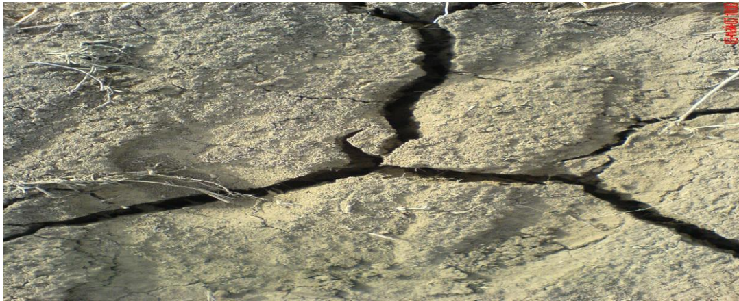
Figure 1. Cracks on the surface of soil
